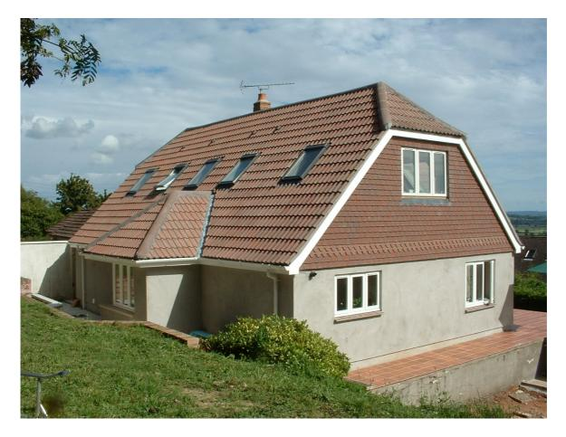
This 1970s bungalow was taken down to it's newly insulated ground floor and walls and rebuilt with rooms in the roof. Highly insulated Timber-frame first floor & Solar Water heating with large windows to the south to maximise solar gain and take advantage of the views across the Levels.
