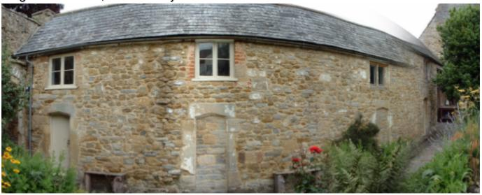
The Chapel and Almshouses (originally the Hospital), date back to the 12<sup>th</sup> century. We strengthened the unsupported Hospital gable, replaced the boundary wall, and replaced all of the damaging cement render and pointing with lime. The site is a Listed Building and Scheduled Monument, and is a much loved and visited site which we were delighted to help bring back into use, including helping to raise the necessary funds from multiple donors.
